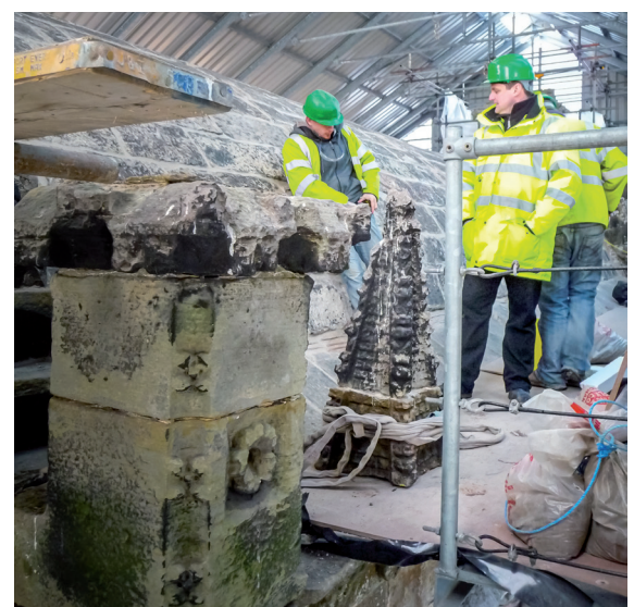
Pinnacle removed for repointing
